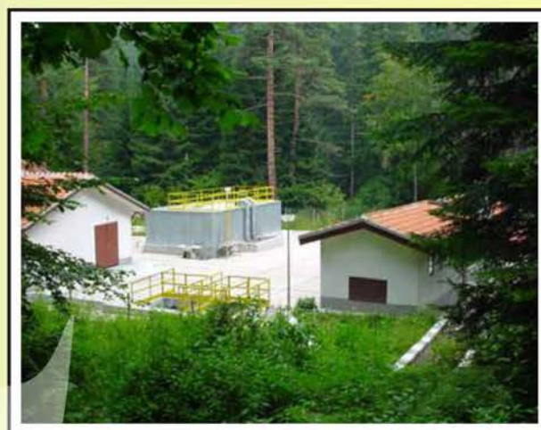
Waste water treatment plant in Borovets resort – 300 000 BGL
