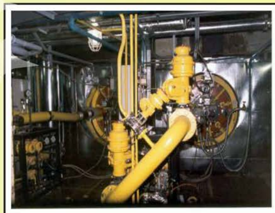
Sofia – East Thermal Power Plant – replacement of the old burners with new, low-nitrogen ones – 2 049 443 BGL (Co-financed by the Danish Environmental Protection Agency)
