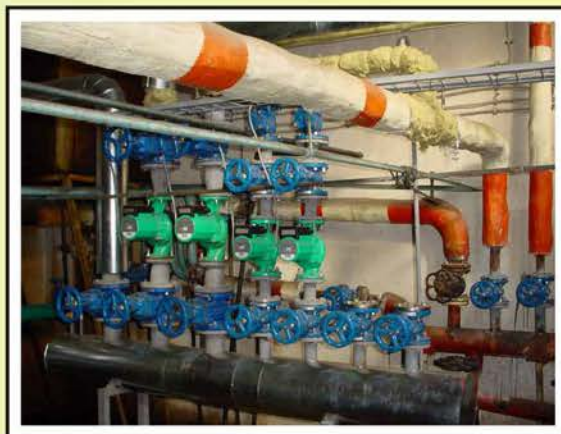
Reconstruction of the heating plants of municipal buildings in the town of Sapareva Bania – conversion from liquid fuels to geothermal energy – 114 827 BGL
