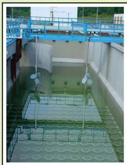
Main sewerage collectors IV and V in the town of Byala, delivery collector, and equipment for the Obzor-Biala Waste Water Treatment Plant – 800,000 BGL (Co-financed by Danish Environmental Protection Agency)
