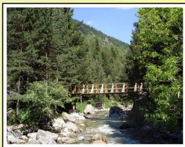
Construction of a tourist trail along Beli Iskar river valley in Rila National Park – 108 439 BGL
