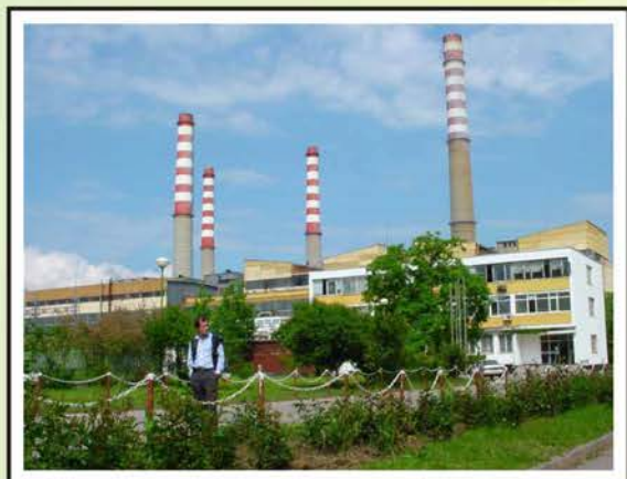
Low-nitrogen burners for boilers No. 5, 6 and 7 of Sofia-Iztok thermal power plant – 2 049 443 BGN
