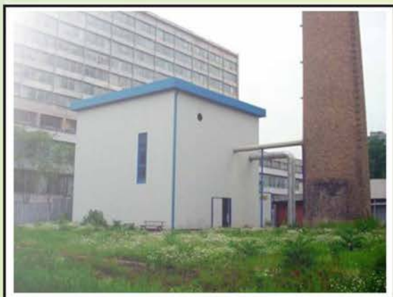
Purchasing and delivery of installation for purification of the gases, released from the incinerator for clinic and domestic wastes at the Military Medical Academy – Sofia – 976 836 BGL
